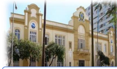
Former Customs Building
